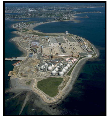
The MWRA Deer Island Treatment Plant, serving Boston and area communities (MWRA photo).
